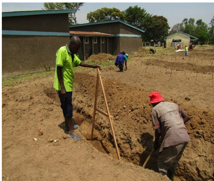
Parents making swales for water harvesting and storage in the soil to boost food production in St Denis school garden
