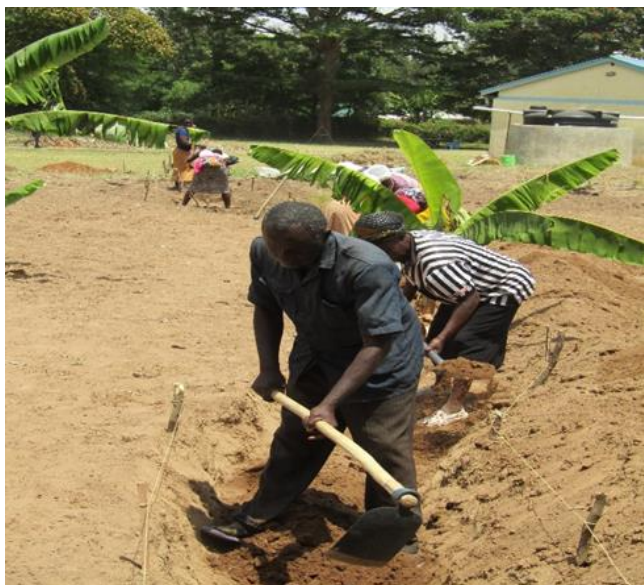
Parents excavating swales for water harvesting.
